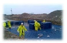
reducing land take. As an attenuation/storage system, tanks are generally used in combination with other SuDS approaches including treatment components. Regular maintenance of attenuation tanks is an important consideration as any failures or blockages are less visible.
