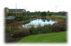
and amenity benefits by supporting emergent and submerged vegetation along the waterline and within shallow marshy areas. Retention ponds need to be designed with suitable upstream pre-treatment systems to prevent open water areas becoming blocked with silt, odorous due to pollution or stagnant. Well managed ponds and wetlands can add significant economic value to a development.
