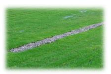
on groundwater levels being at least 1 m below the base of the feature and soils having a suitable permeability. Infiltration to the ground at or near the source reduces reliance on downstream drainage systems.
